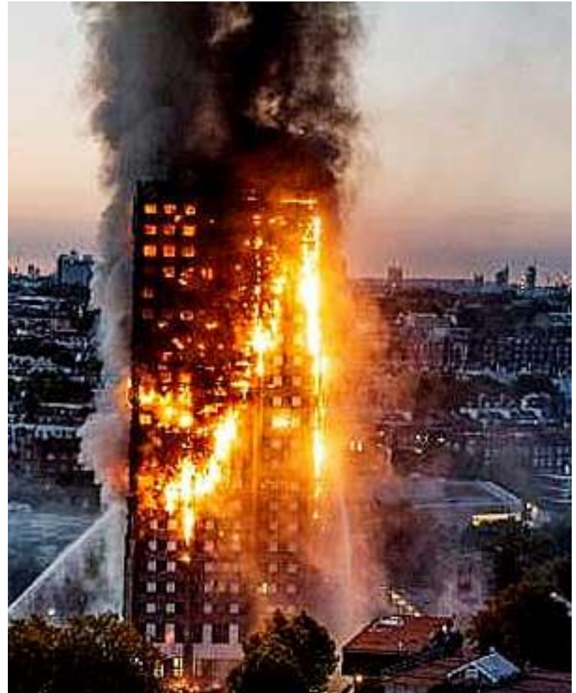
Source: freemalaysiatoday.com: 2017 fire at "Grenfell Tower", London
