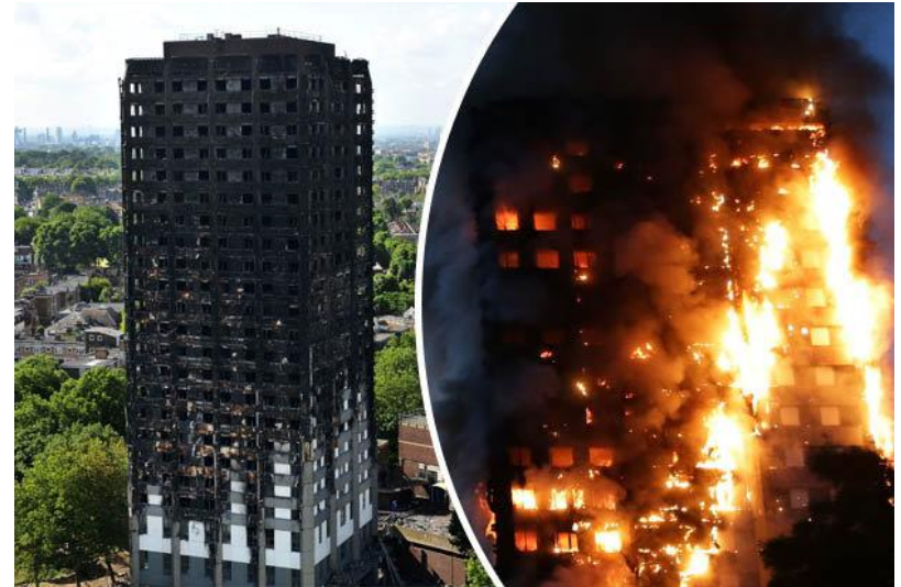
Source: DailyStar.co.UK: 2017 fire at “Grenfell Tower”, London
