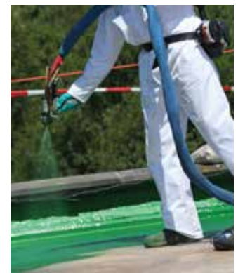
Installation of Prodeq FX400 membrane
